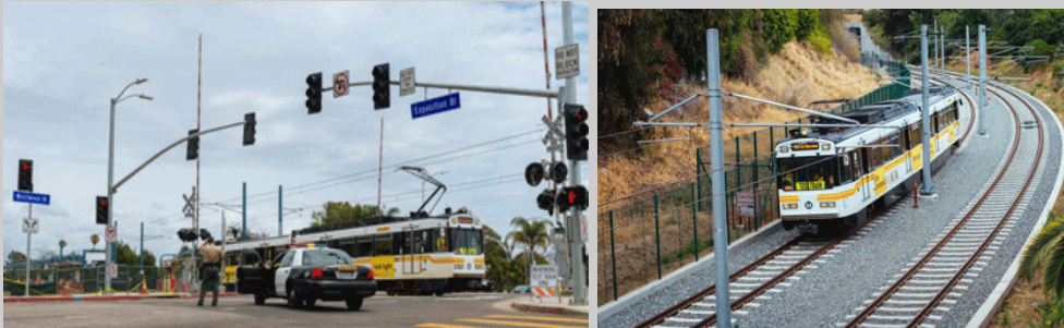
Car 126 on westbound track crossing Westwood Boulevard (left); Car 126 on westbound track in Cheviot Hills (right).
