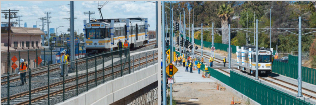
Car 130 just west of the Venice Boulevard Overcrossing westbound (left) 4-7-15, and approaching Bagley Ave. (right).
